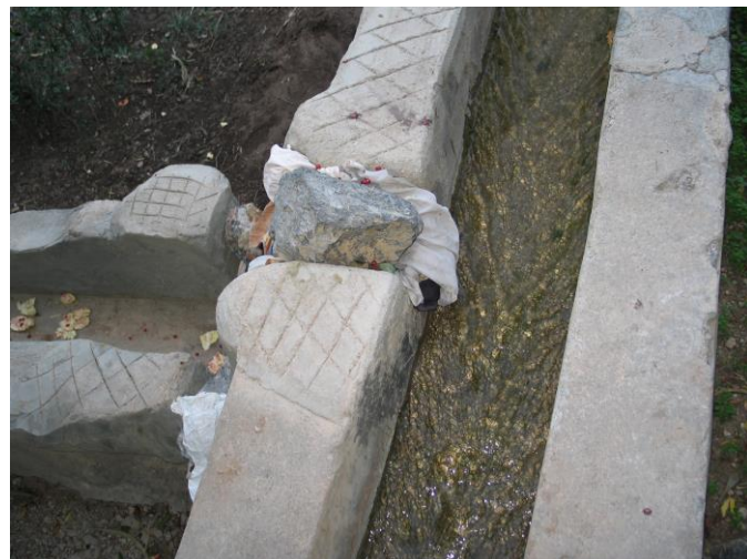
Water Junctions in the Falaj System
