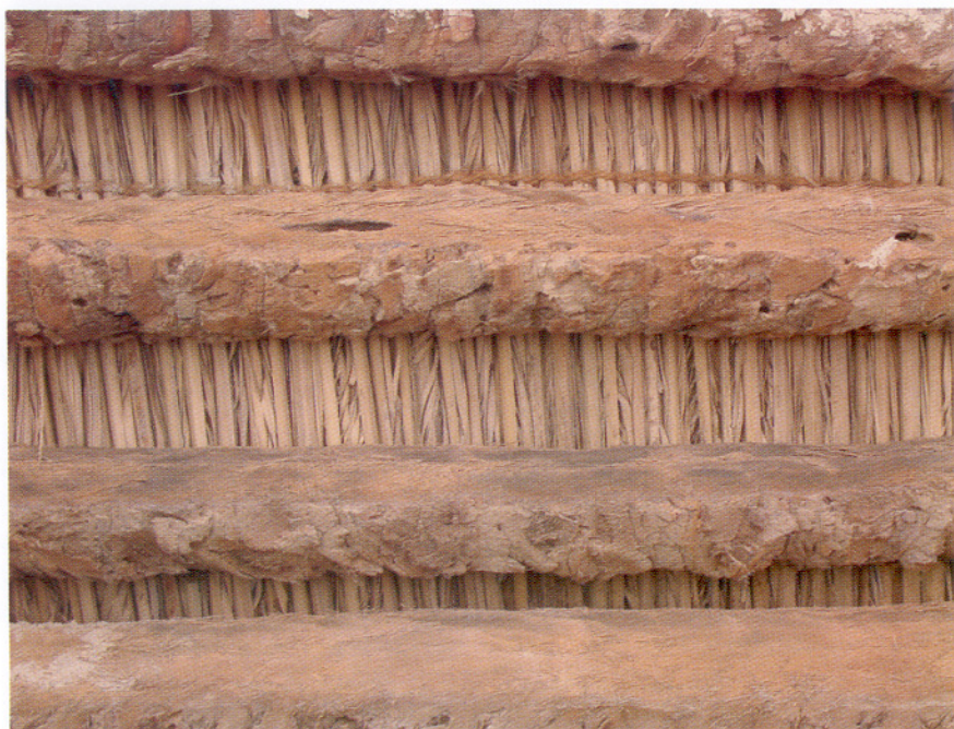
Da'an and split palm logs used to make a roof
