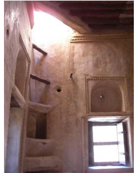
The stair to the viewing level
