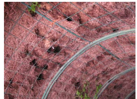
House sparrow nests in the roof of the arbour
