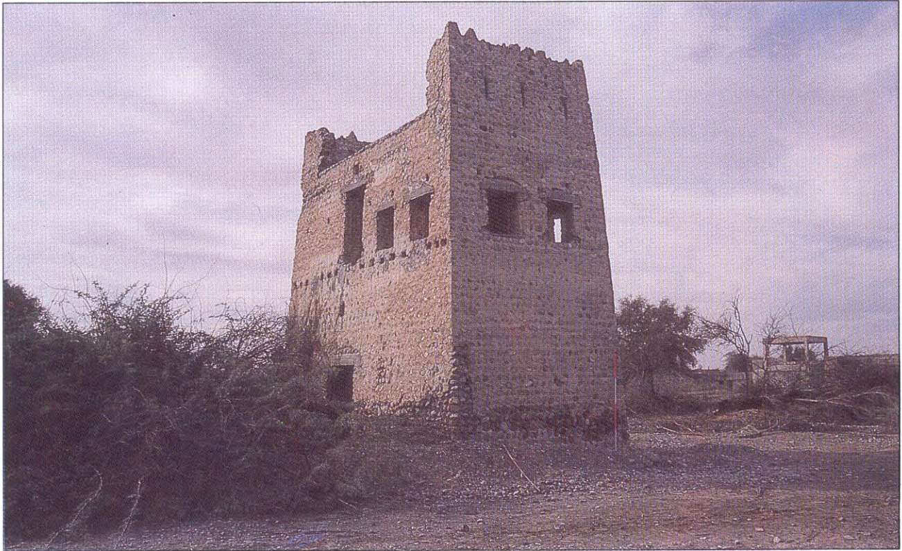
The house-tower at Falayya, Ras al Khaimah, built of cobbles and mortar. One of the best surviving examples of a Type 1 Tower.
