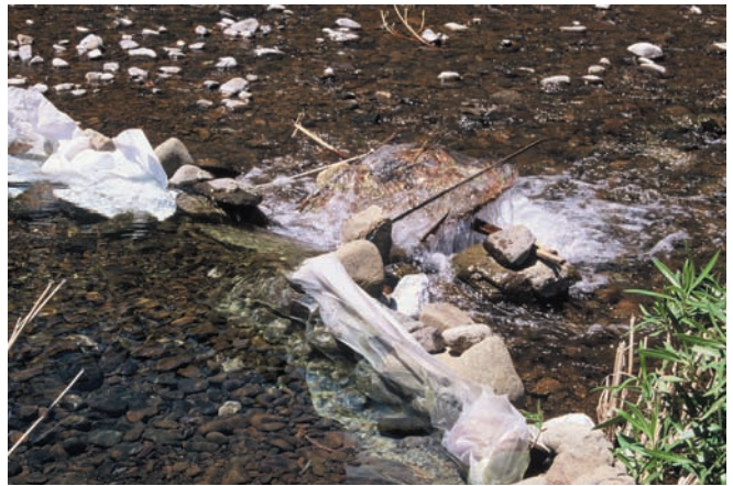
Fig 2. A plastic-lined dam and 'weir' in Wadi Qahfi, now neglected but recently used for fishing
