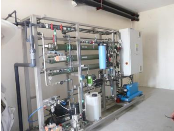
Electrical system panel at the Oryx Center Photo: May Yoke Taylor
