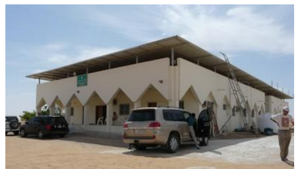
Arabian Oryx Protected Area HQ Building Photo: May Yoke Taylor
