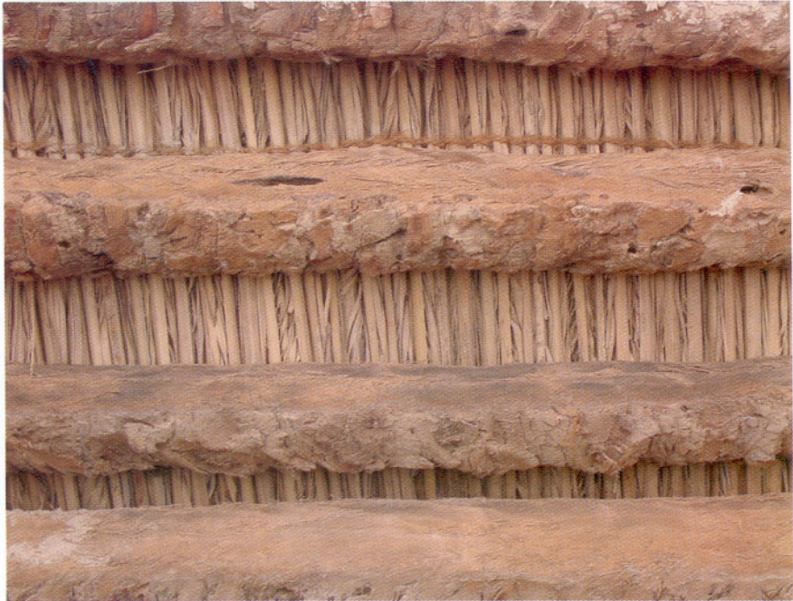
Da'an and split palm logs used to make a roof
