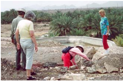
Checking the plumbing
