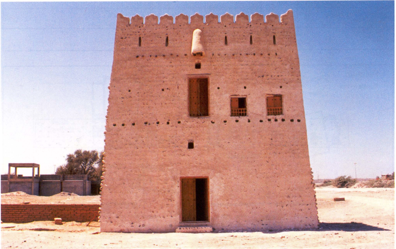
Plate 2: The restored stone tower
